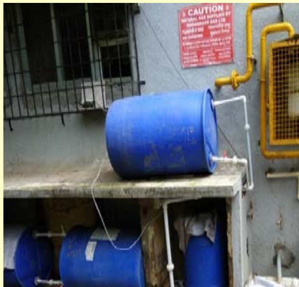
Photo: Grey Water Treatment System
